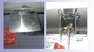
This solution prevents access to the release lever by thieves while leaving the lever fully operational so that the door can be opened manually in case of a power outage or fire.
